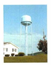
Coolfont Ridge Storage Tank – The project involved a booster station, 10,000 linear feet of sewer line, 28 manholes and 12,000 linear feet of waterline. Another portion of the project involved the planning, design and construction phase services for a 67,000 gallon storage tank.
